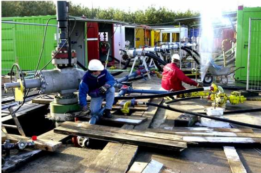
Hydraulic testing at Horstberg.
